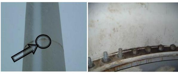
Crack in the weld of the tower
